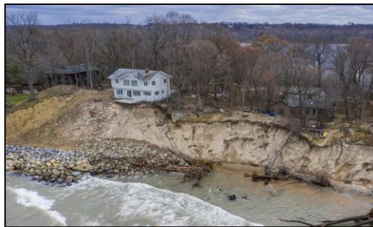
Shoreline Erosion- near Stevensville, MI
